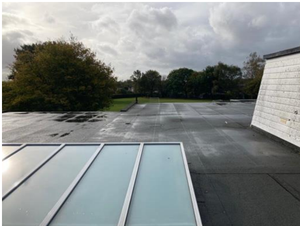
Solar panel present on the roof
