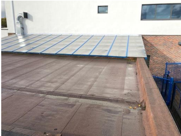
Overview of roof E
