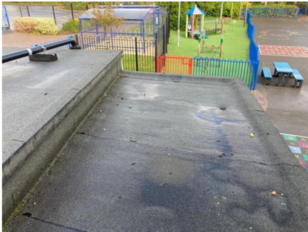
Overview of the roof area
