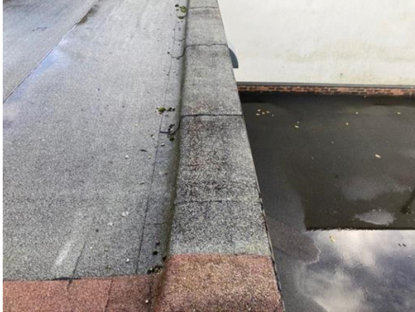
Overview of perimeter kerb
