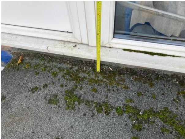
Window cill circa 120mm above the roof surface
