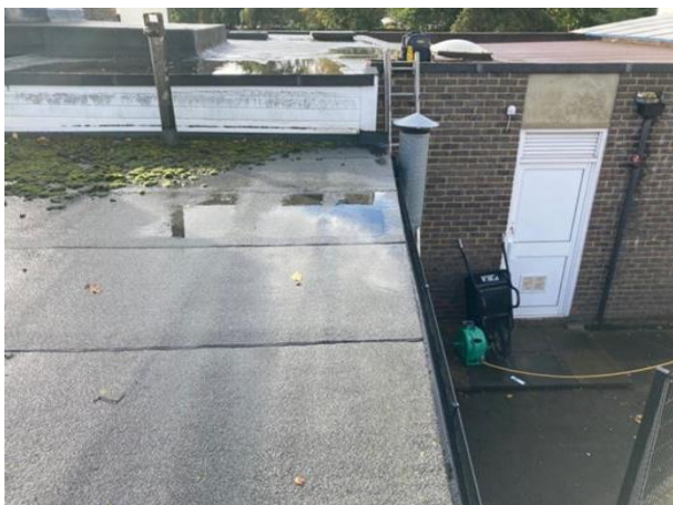
Overview of the roof area
