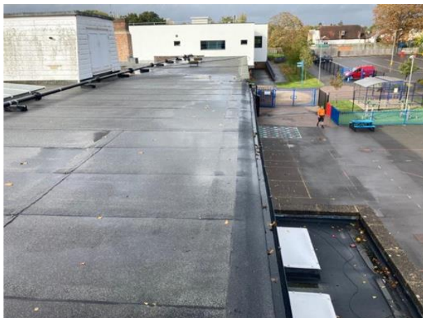
Roof drains into external gutter
