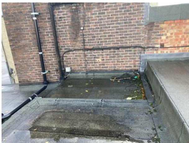
Overview of the roof area
