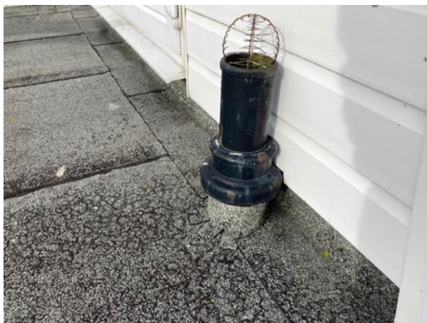
Soil vent pipe near the UPVC cladding
