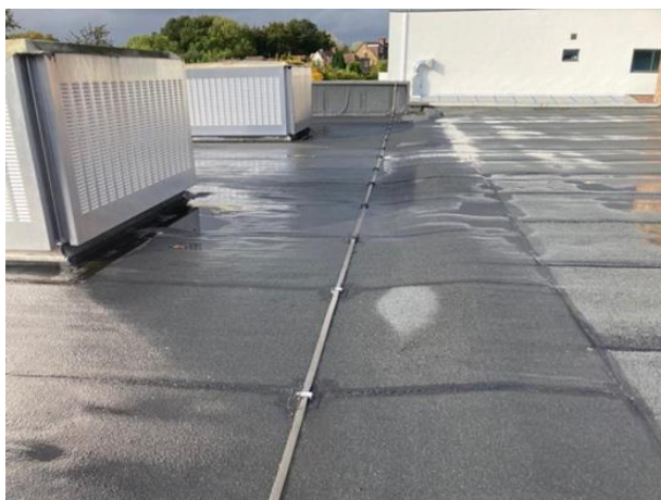
Overview of the roof area
