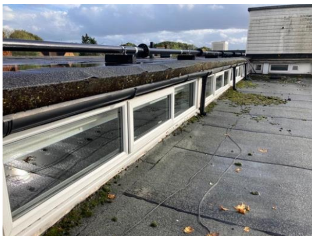
Overview of windows
