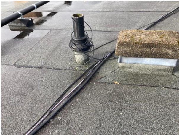
Soil vent pipe present on the roof
