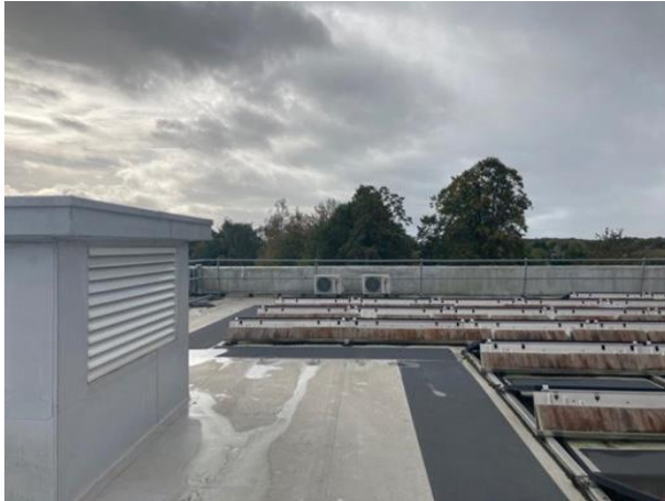
Overview of the roof area
