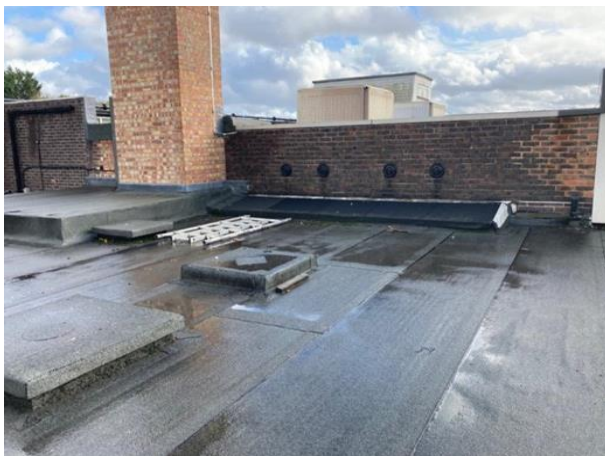
Further overview of the roof area
