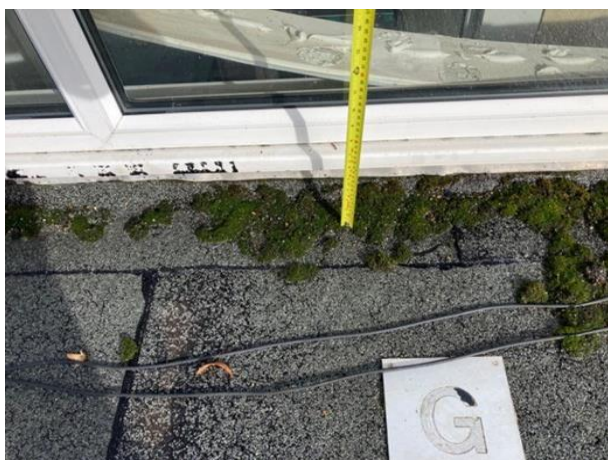
Window cill circa 130mm above the roof surface
