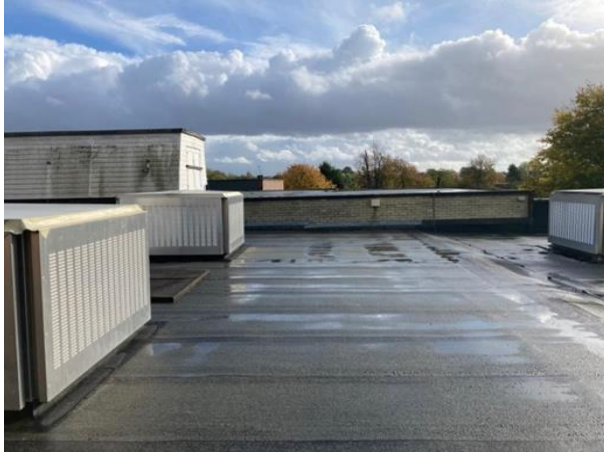
Overview of the roof area
