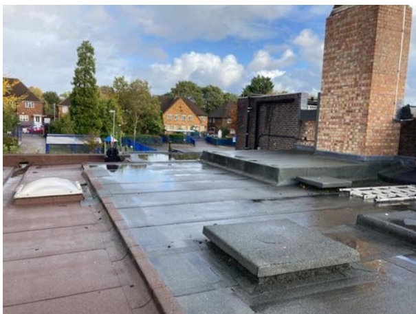
Overview of the roof area
