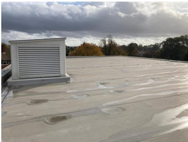
Overview of the roof area
