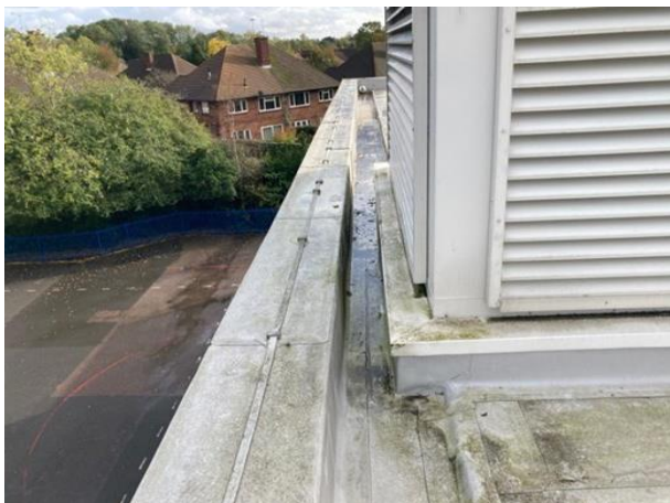
Further overview of the roof area
