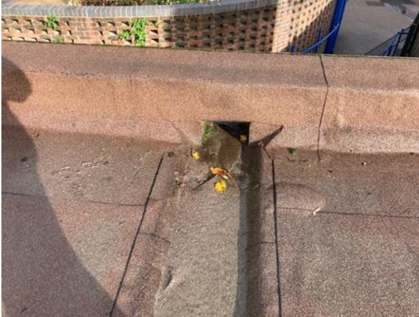
Overview of internal gutter
