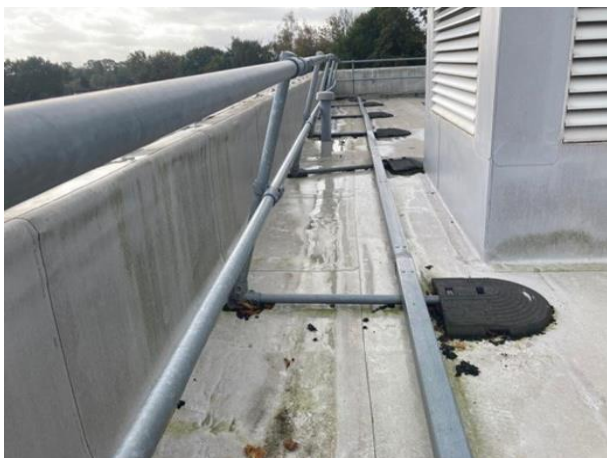
Handrail present around the perimeter
