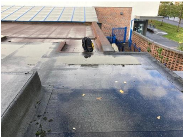
Overview of the roof area
