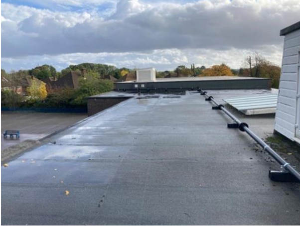
Overview of the roof area
